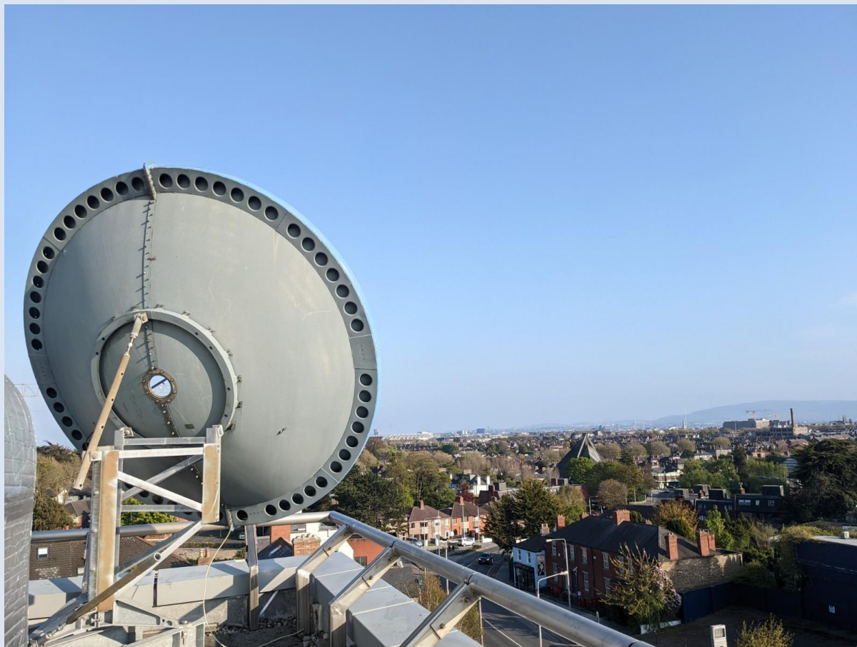
Figure 12 3M dish Met Éireann use to access the weather satellite
