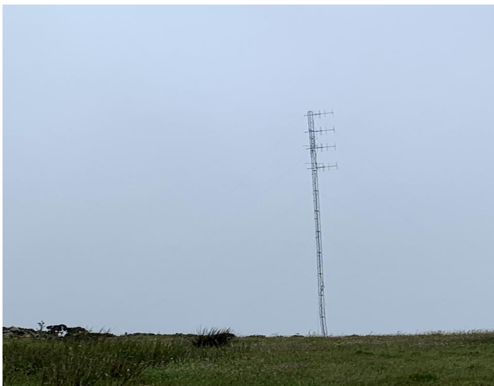
Figure 15. Unlicensed transmitter site
