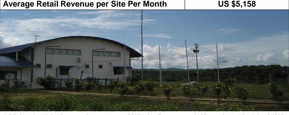
Kalabakan, East Malaysia supporting an average of 252 subscribers per month. Picture shows 1.8m C-Band VSAT backhaul antenna with 1.2m GSM omni antenna mounted on a 12 metre mast with lightning protector. 37dBm booster provides a coverage radius of  $\sim$  5km
