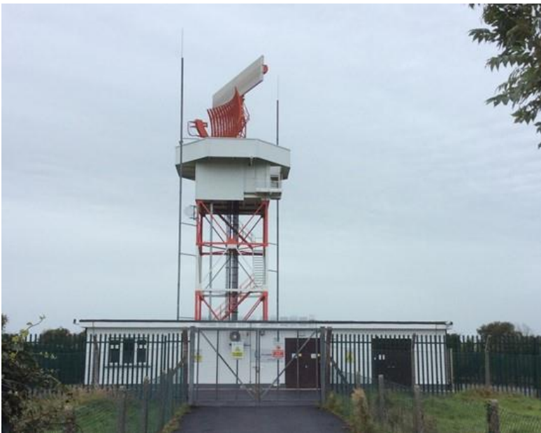
Figure 1.1: S-band radar (STAR2000) at Shannon
