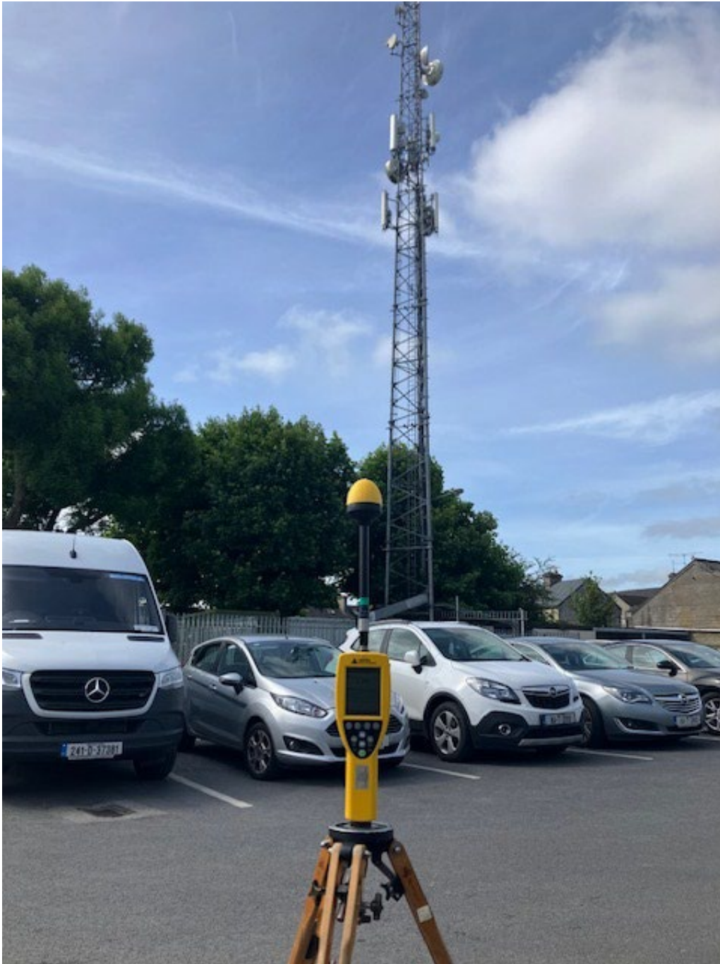
Photo 1. Broadband Measurement location looking towards antennas
