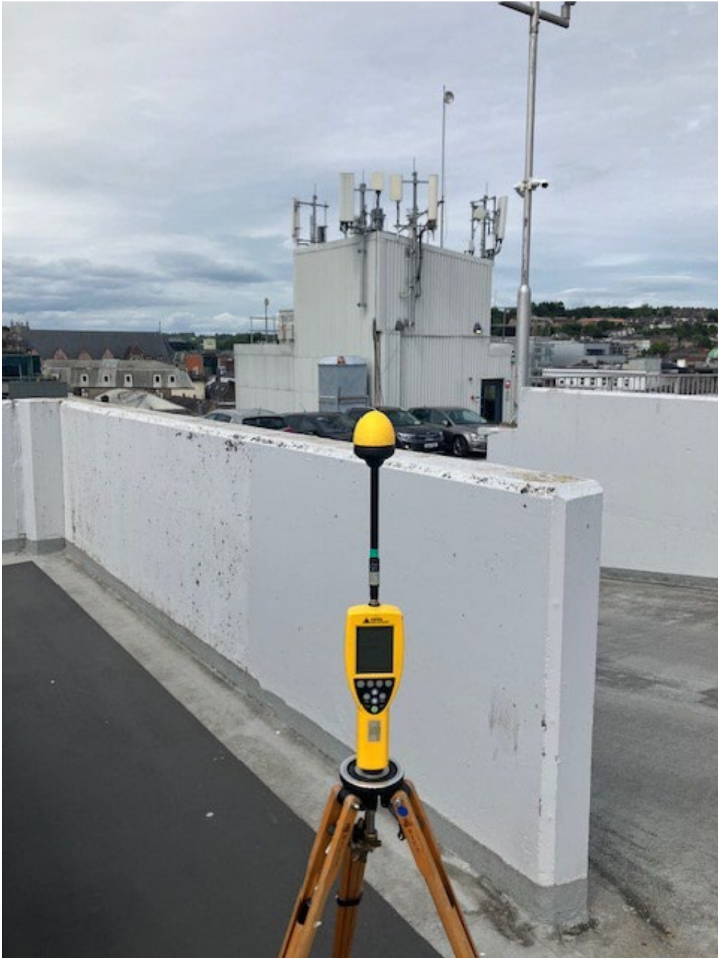
Photo 1. Broadband Measurement location looking towards antennas
