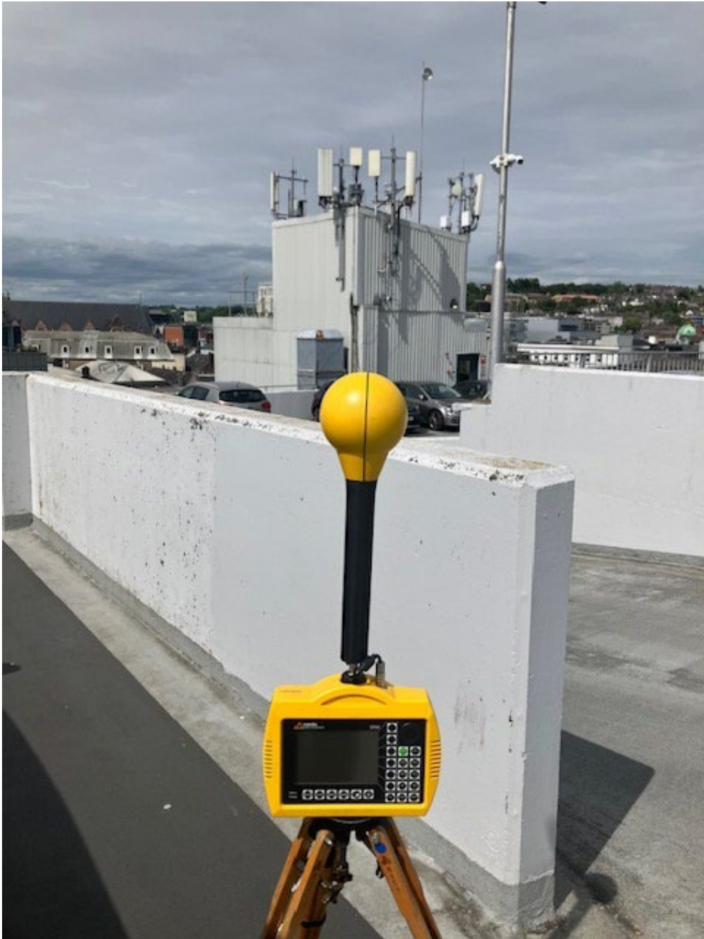
Photo 2. Frequency selective measurement location looking towards antennas
