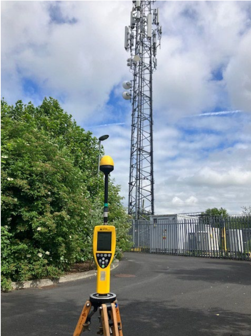
Photo 1. Broadband Measurement location looking towards antennas
