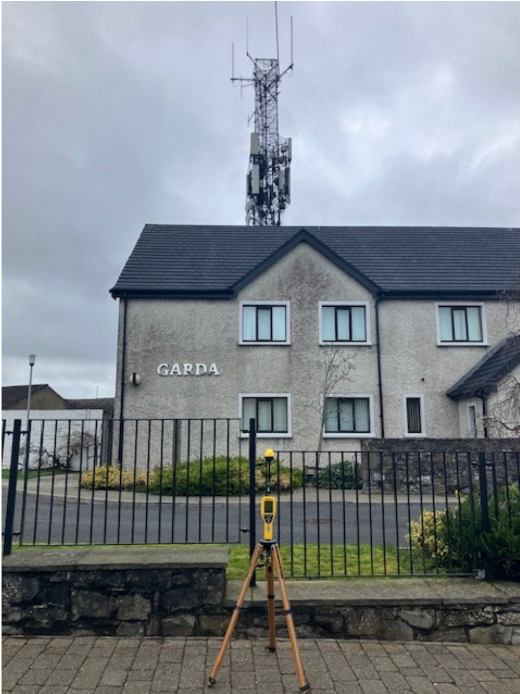
Photo 1. Broadband Measurement location looking towards antennas
