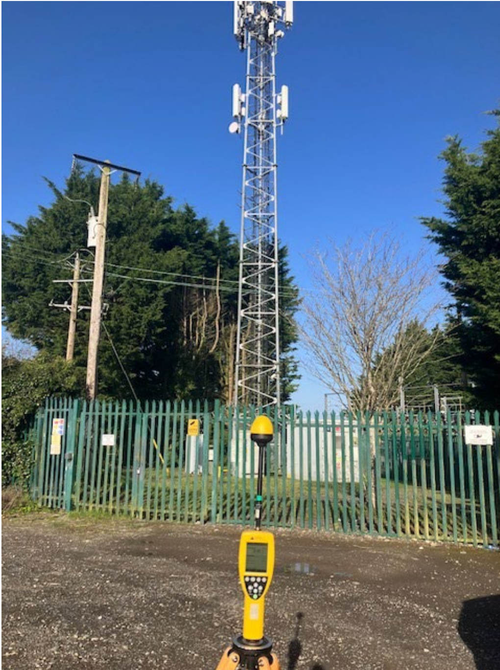
Photo 1. Broadband Measurement location looking towards antennas
