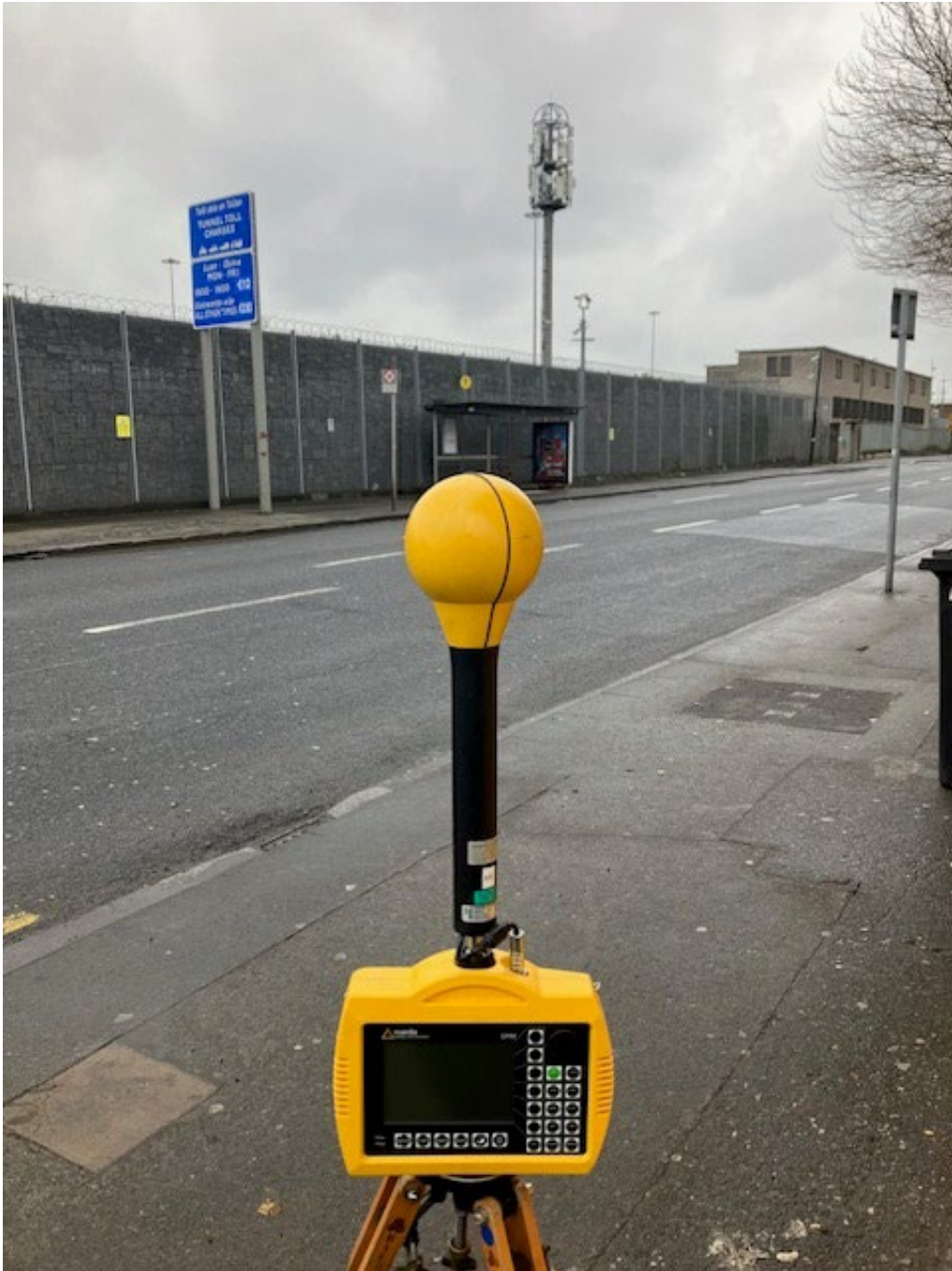
Photo 2. Frequency selective measurement location looking towards antennas
